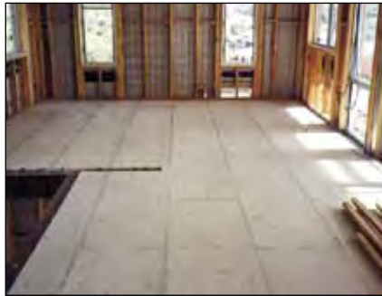
Fig 1.2 Residential Suspended First Floors
