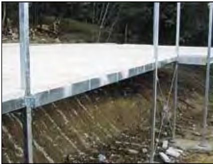
Fig 1.1 Residential Suspended Ground Floors
