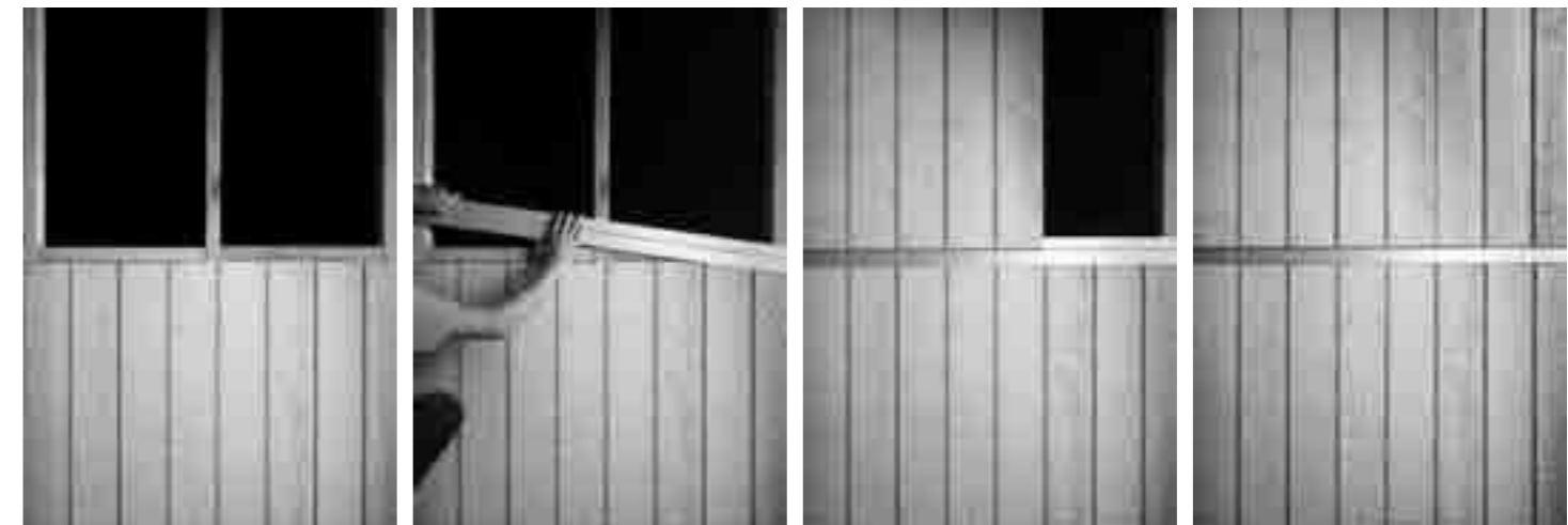
Note: Weathergroove Woodsman shown. Direct fix method shown. In the interest of clarity cavity fixing method and vapour permeable sarking have been omitted.
