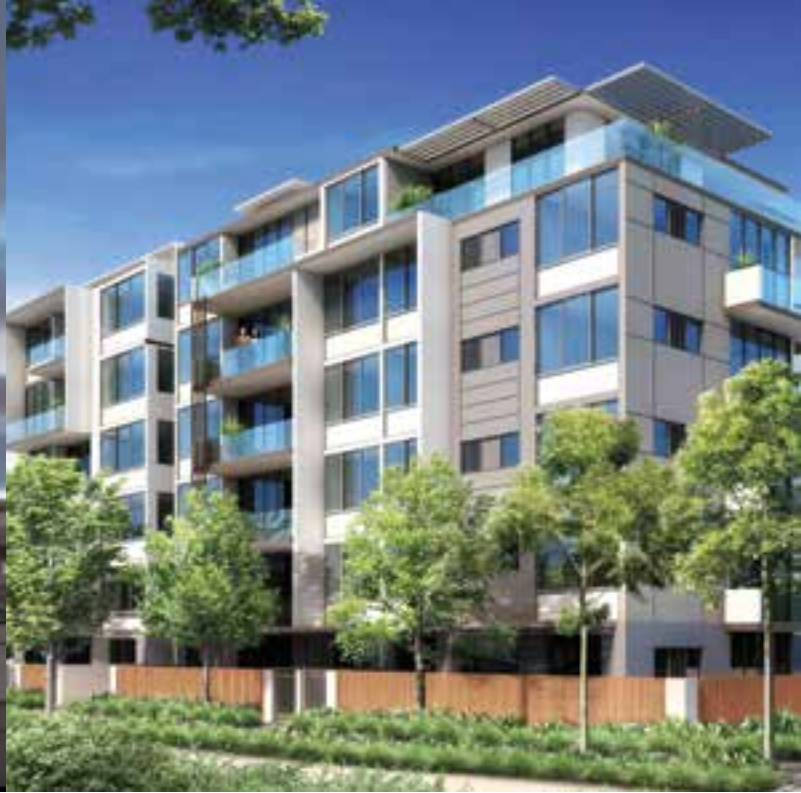
Epping Park by Meriton Apartments.
